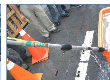
Injection pipe with double packer (inner pipe)
