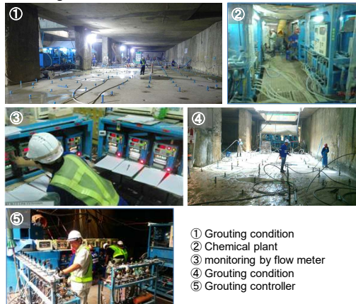
Injecting a sealing grout, inserting a outer pipe
