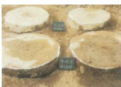
EX-DJM (拡大径翼杭施工)
