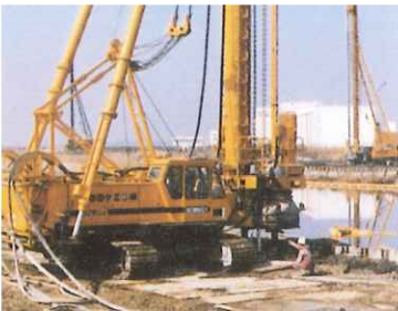
護岸背面の改良補強 (DJM2070) Job site on revetment work
